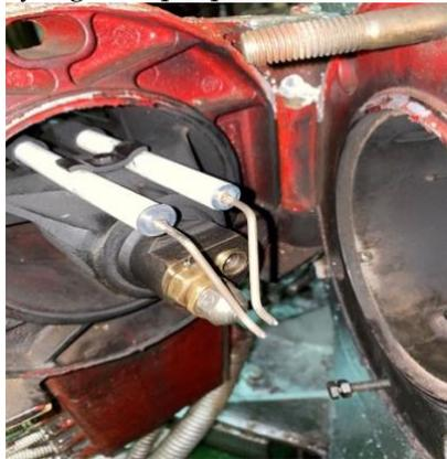
Gambar. 6 *Electrode Burner Boiler*
