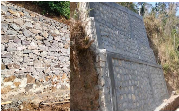
Gambar 1. Dinding Gravitasi ( Gravity Wall )(Febrialdi, Tanjung, and Hasibuan 2022)
